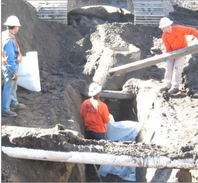
Figure 2 Shoring a Step-Trench
