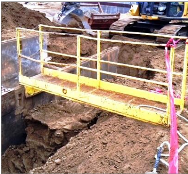
Figure 2 Shoring a Step-Trench
