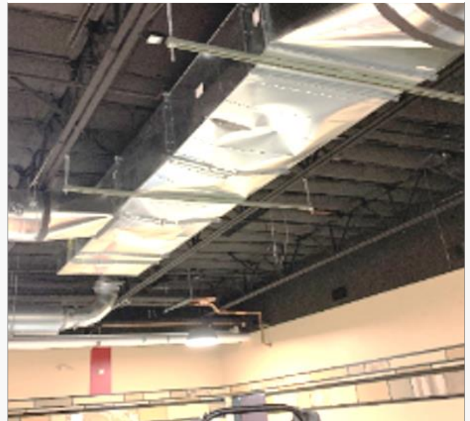
ENTIRE DUCTWORK PRESSURE COLLAPSE
