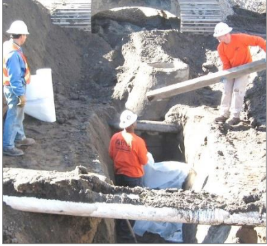
Figure 2 Shoring a Step-Trench
