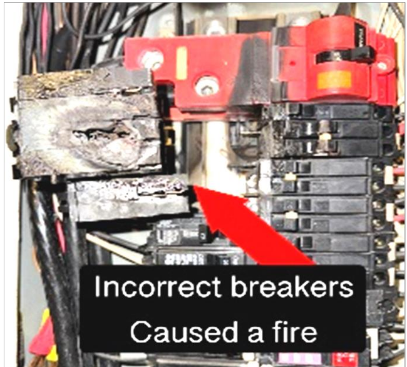
Burned Breakers
